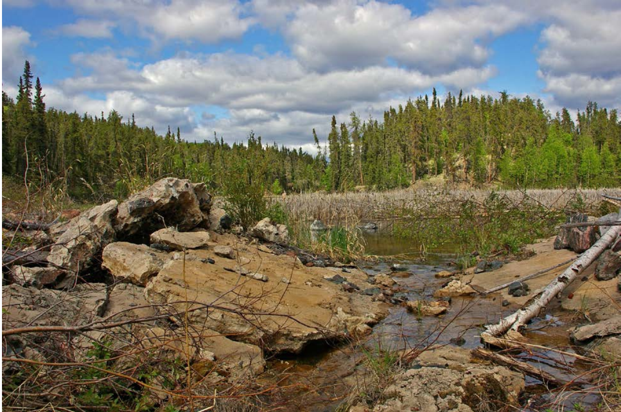
Photo 3 – Ice-jacked block on north side of Marie Spillway
