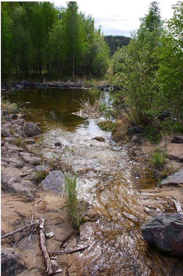
Photo 2 – Marie Reservoir Spillway (water flowing into stilling basin)
