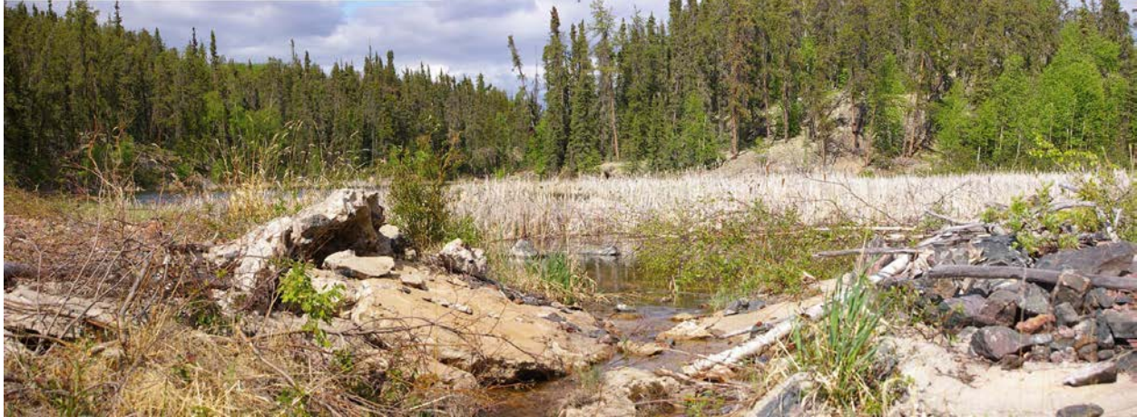
Photo 1 – Marie Reservoir Spillway looking upstream
