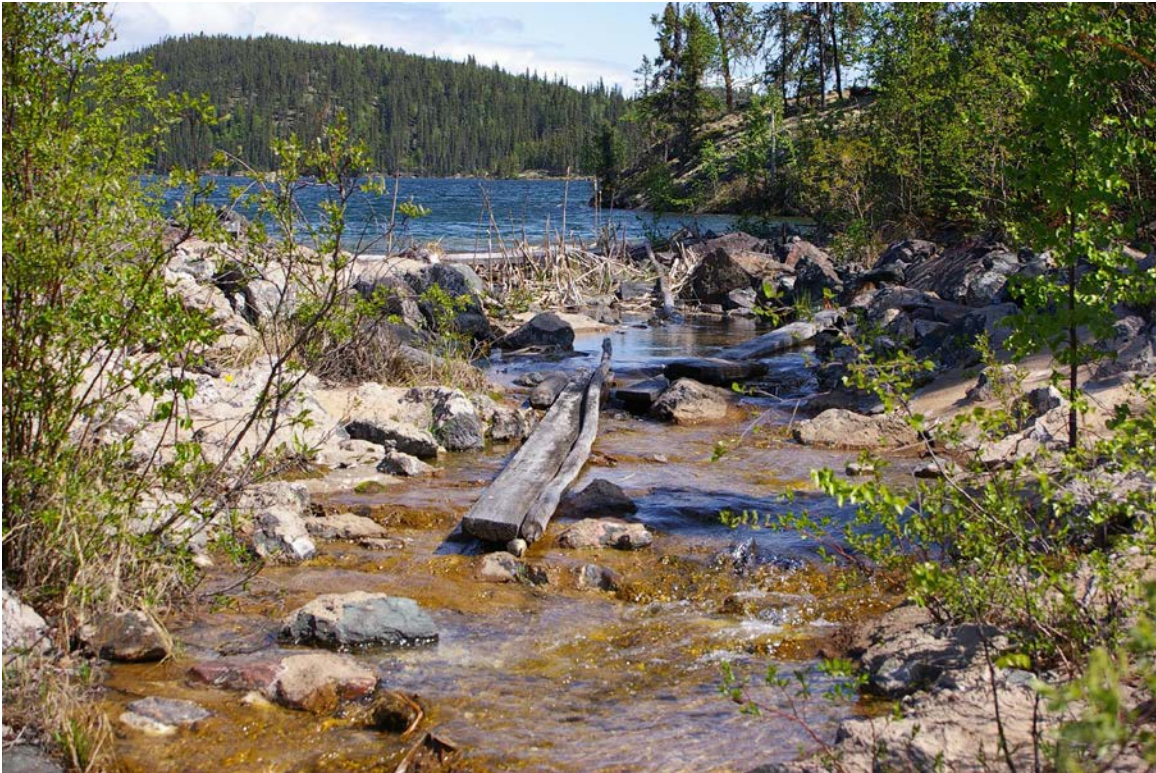
Photo 4 – Fookes Reservoir Spillway looking upstream
