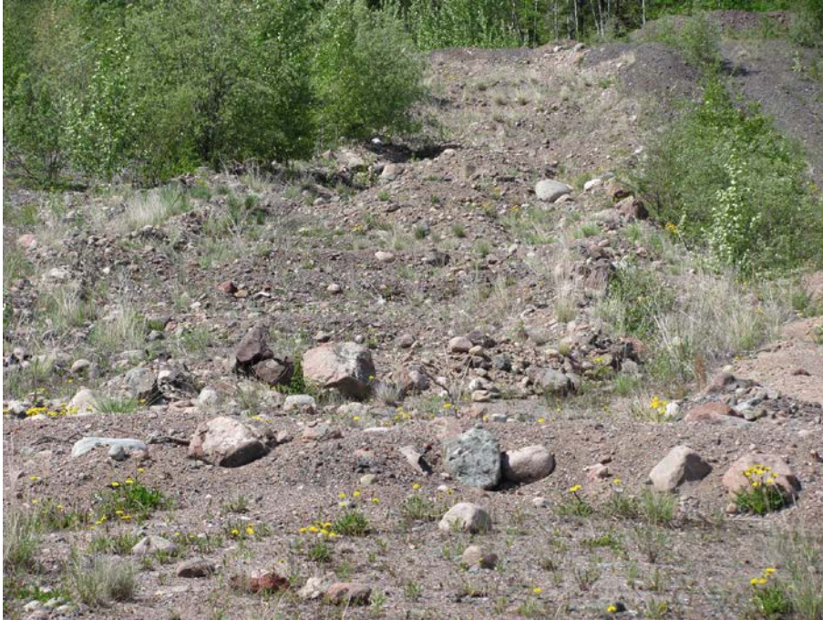
Photo 10 – Chevrons in place on north access point to the Fookes delta
